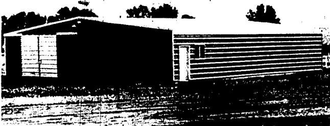
A NEW ADDITION to the Dixon County Fair grounds is this all-metal building built by the Dixon County Agricultural Society. The building was used for Pre-Fair Day Tuesday and also will be used for square dancing and teen dancing during the Dixon County Fair next week.
